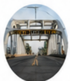
Edmund Pettus Bridge (Selma)
